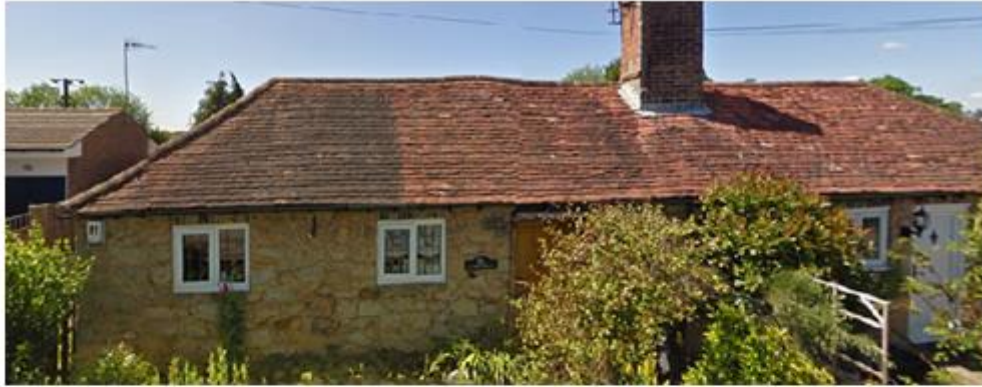
Crowhurstland Dairy Cottages West Street above
